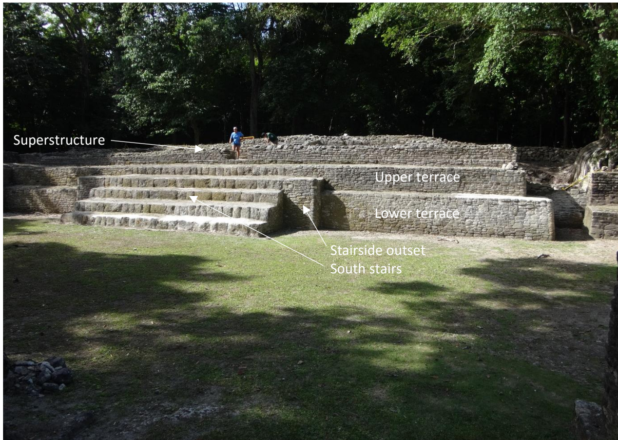
Figure 6.2. The south side of Structure N10-15 as seen from across the courtyard indicating some of the architectural features to be discussed in this chapter (photo by Karen Pierce, 2014).
