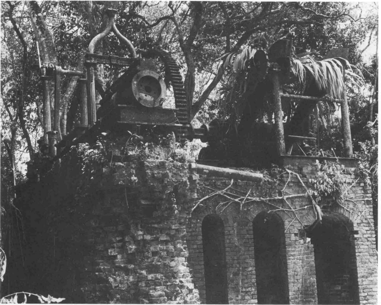
Figure 5. View of the mill from the southwest, showing the relationship between engine and crusher. Note the steam supply pipe extending to the right of the engine.
