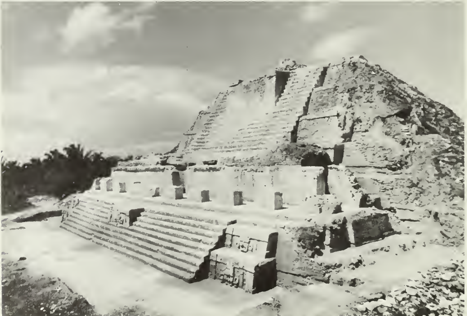
Plate 6 A stair block of standard size graces the lower stair of this structure; the upper stair boasts one of the more massive examples of a stair block. The lower block resembles the stair-side outsets in the foreground in that it possesses both a cornice or superior moulding and façade-sculpture adornment.
