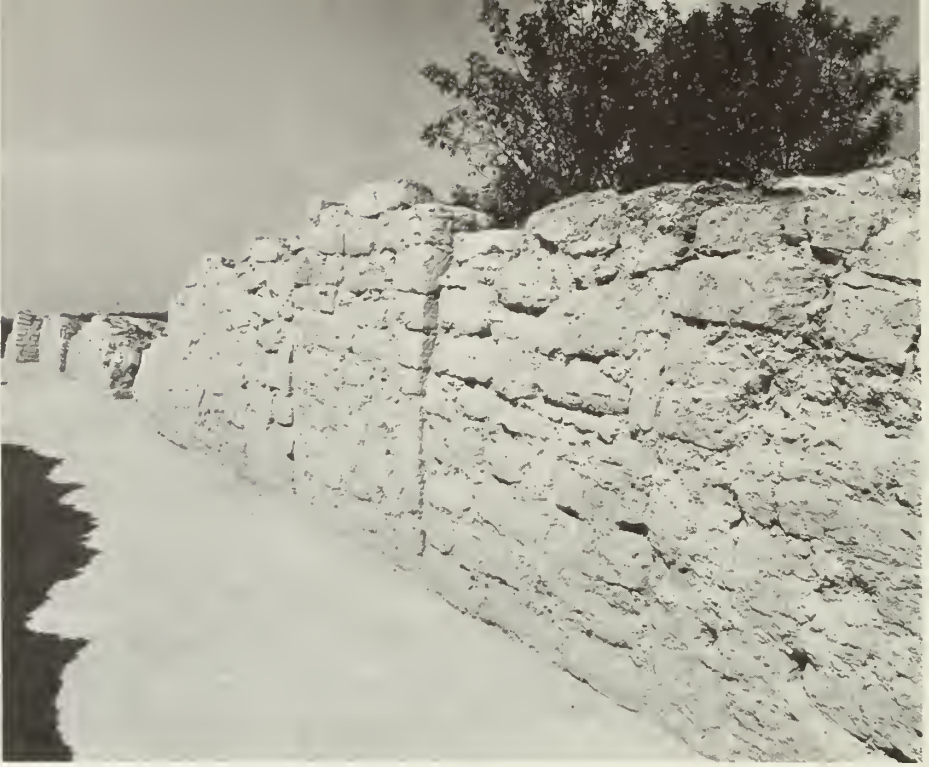
Plate 5 Doorways, many of them sealed by secondary units of masonry. Between the doorways are wall piers almost identical in width to the entryways themselves.
