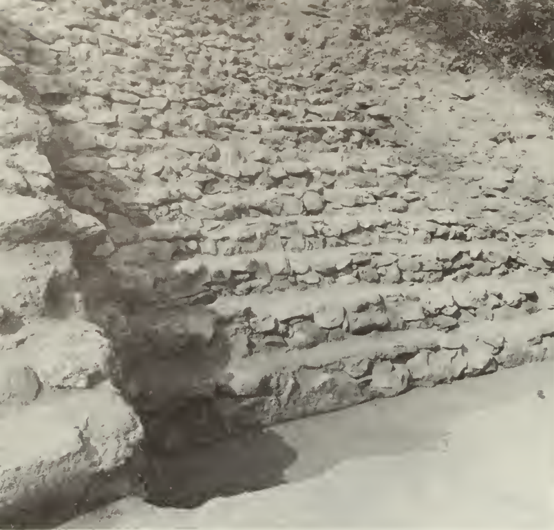
Plate 1 Section through a stair face and backing masonry, showing a core face that duplicates the form of the façade.
