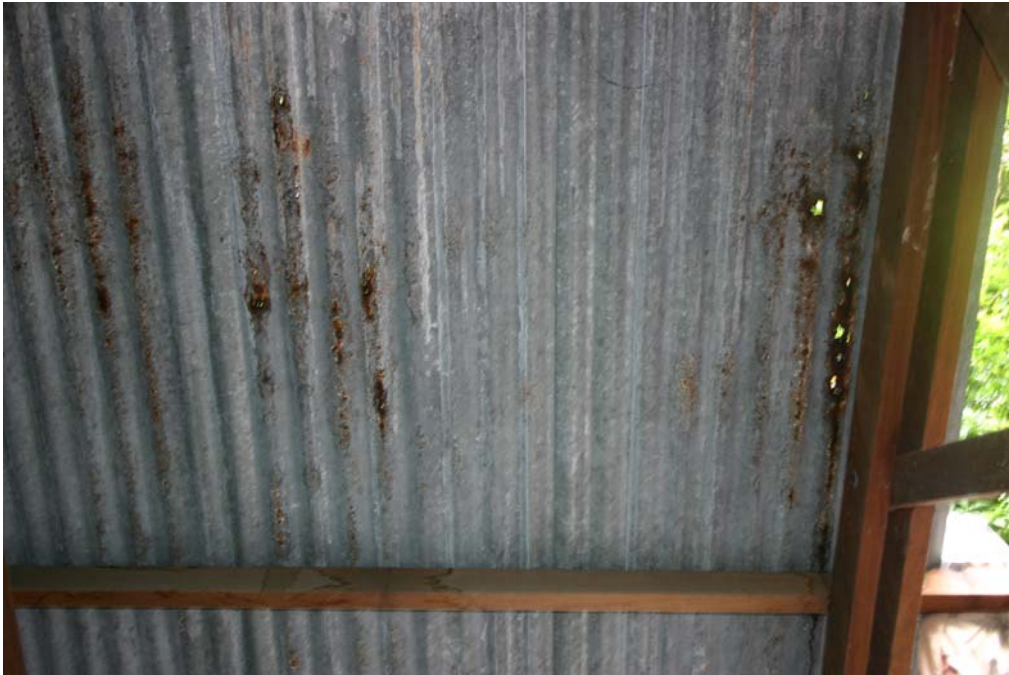
Figure 4: Photograph of the interior of the Museum roof showing an extensively corroded panel containing numerous large holes just prior to replacement.
